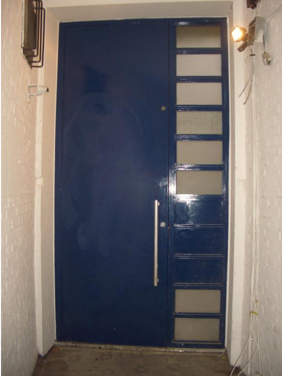
Entrance system before
